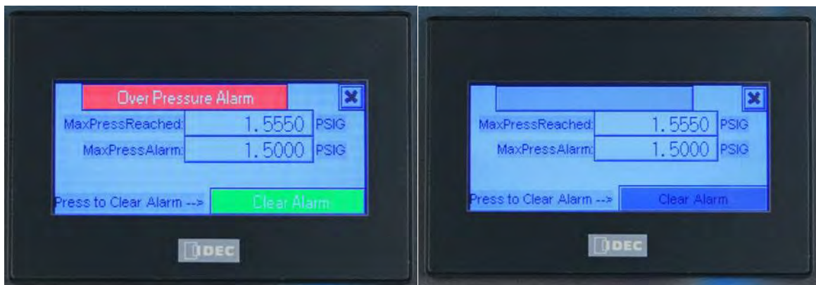
Figure 23 – Max Pressure Alarm
